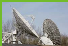
Base Stations BTS
